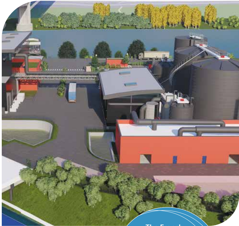
The anaerobic digestion plant in Gennevilliers will transform biowaste from the Paris region into fertiliser for agriculture and gas, to be fed directly into the local gas network.
