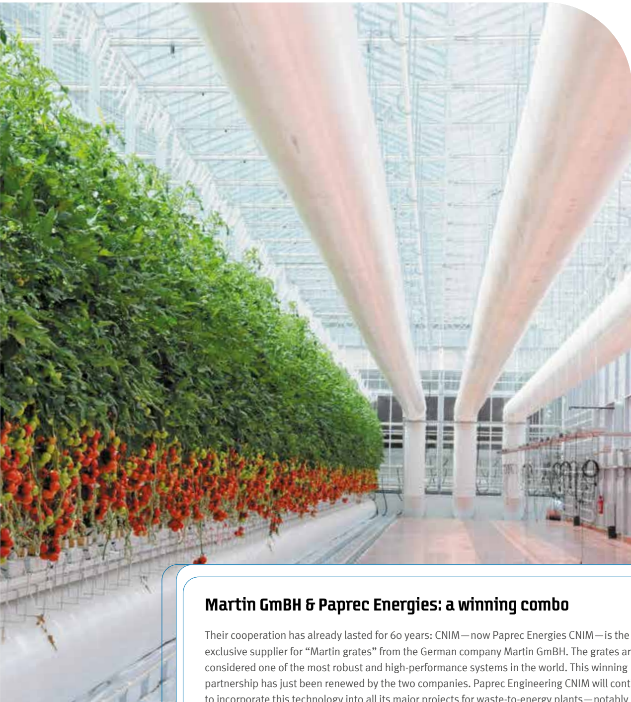
In Pontenx-les-Forges, in south-west France, the WTE plant supplies 80% of the energy needed for heating the Grands Lacs greenhouse, where tomatoes are grown.
