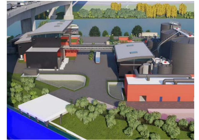
Paris bio-waste methanisation plant
