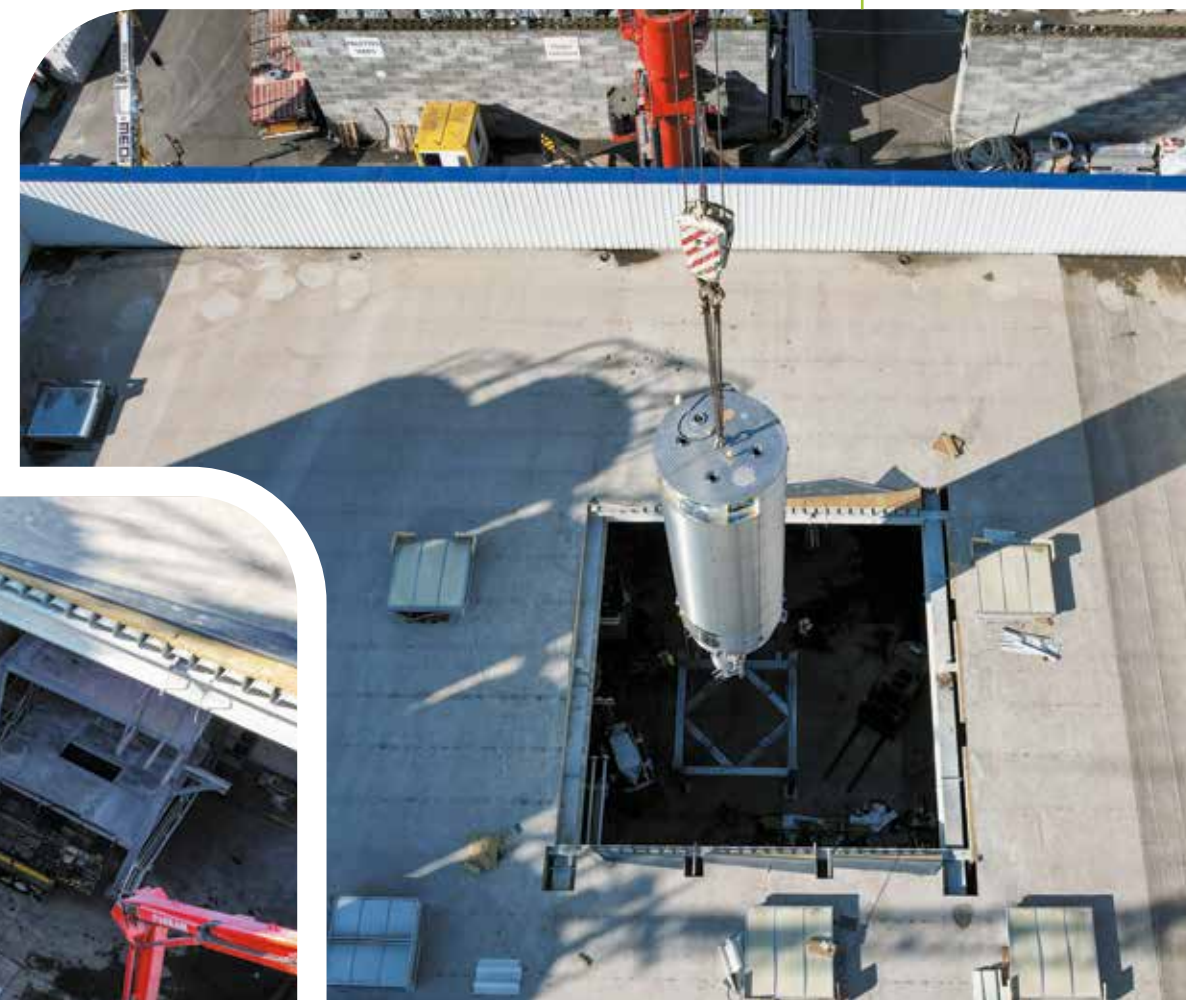
With the help of a mobile crane, the equipment, weighing tens of tonnes, is lowered through the only possible way in: the roof. The installation of a silo is a painstaking operation.
