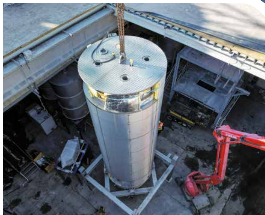
With the help of a mobile crane, the equipment, weighing tens of tonnes, is lowered through the only possible way in: the roof. The installation of a silo is a painstaking operation.
