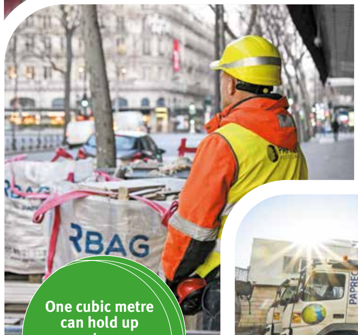
Big bags can also be used to sort waste directly at the construction site and therefore to remove smaller volumes of plastic or cardboard waste.
