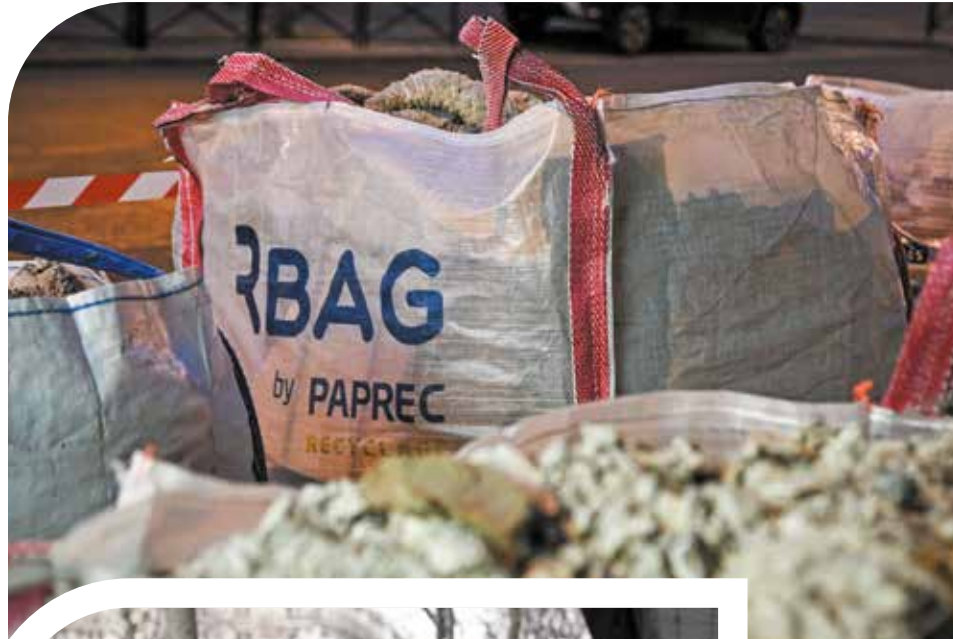
Big bags can also be used to sort waste directly at the construction site and therefore to remove smaller volumes of plastic or cardboard waste.
