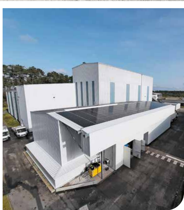
The plant operated by TIRU in Saint-Perdon received the 2021 environmental transition award from the editorial team at L'Usine Nouvelle for its process for using solar energy to produce solid recovered fuel (SRF) from household waste.
