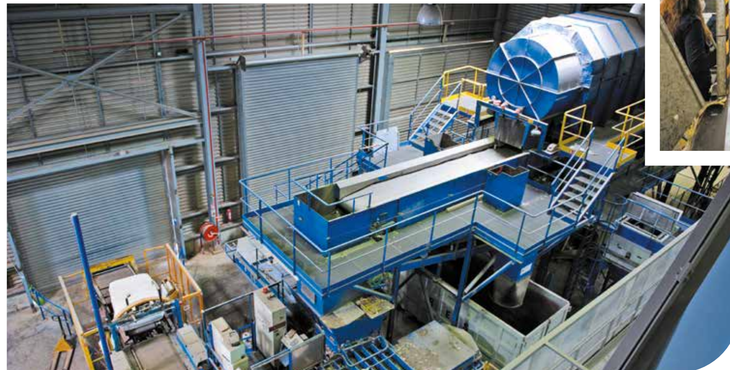
The site in Perpignan has a line for baling waste stored in pits to ensure continuity of service during scheduled shutdowns.
