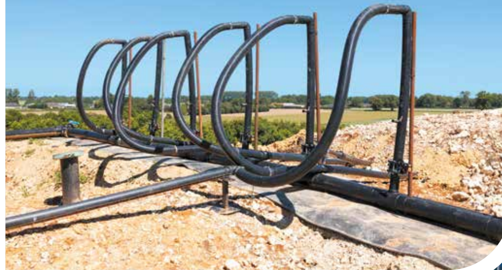
At Paprec's non-hazardous waste storage facilities, the biogas produced from the stored final waste is captured and injected into the grid where it is used to produce electricity and heat.
