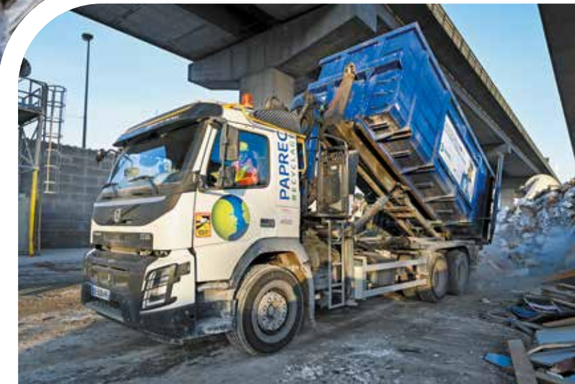
The contents of one cubic metre, which can hold up to 1.5 tonnes of rubble, are emptied at the site. The waste will be sorted and recycled or recovered.
